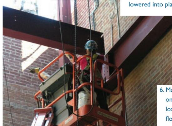
6. Manoeuvring one of the loading gallery floor beams into position.
