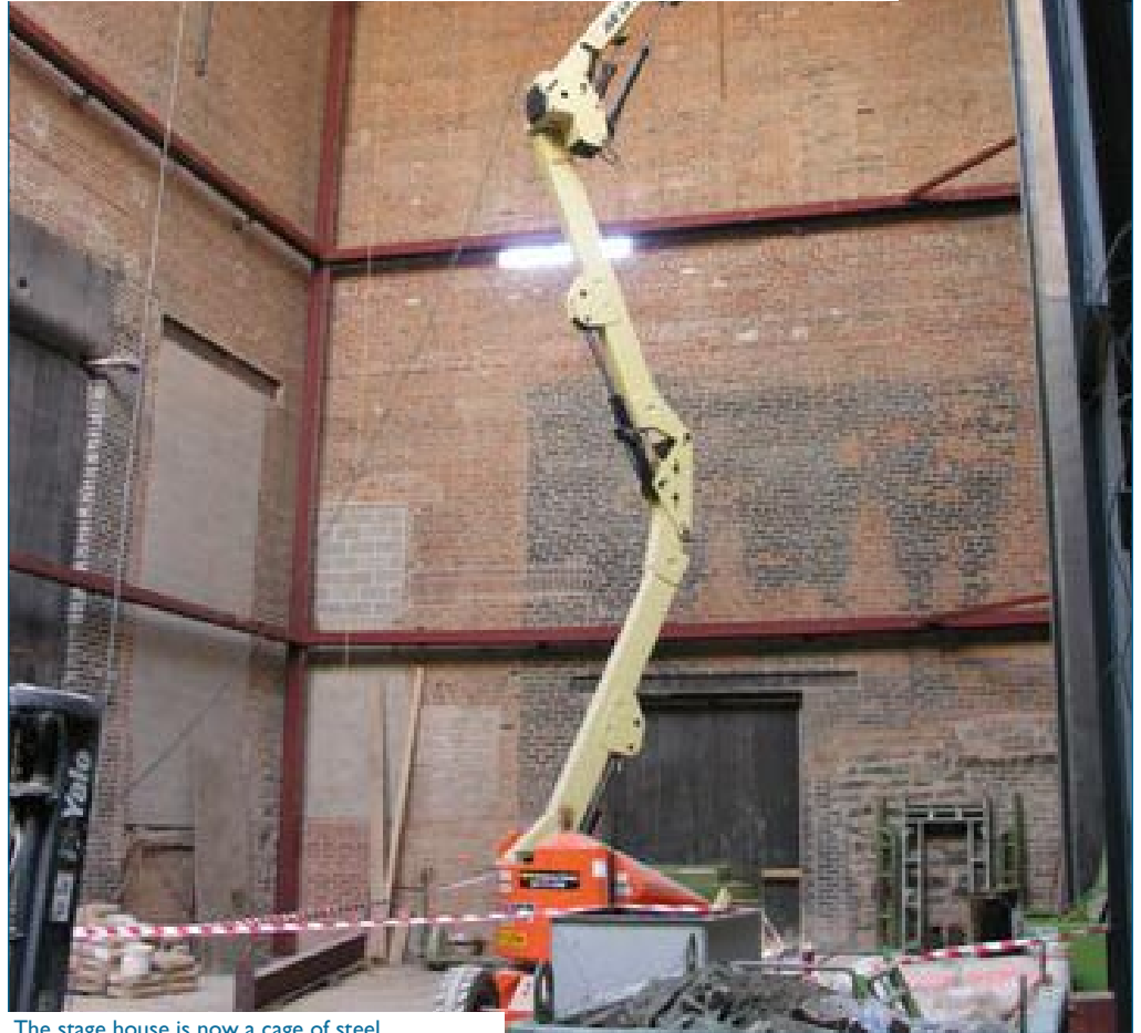
The stage house is now a cage of steel.
