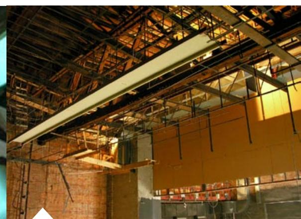
One of the old lighting catwalks in process of demolition. With the ceiling in place these catwalks were slightly less scary, but not a lot...
