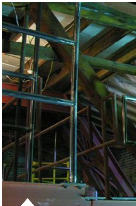
This view showing the catwalk and the rails gives an idea of how these structures also serve as roof trusses.
