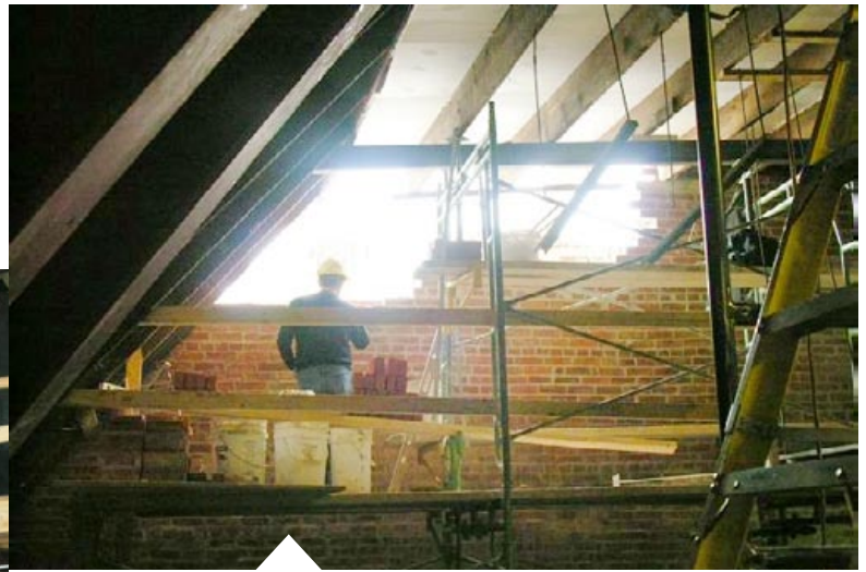
Rebuilding the top of the brick wall- west side of the building.
