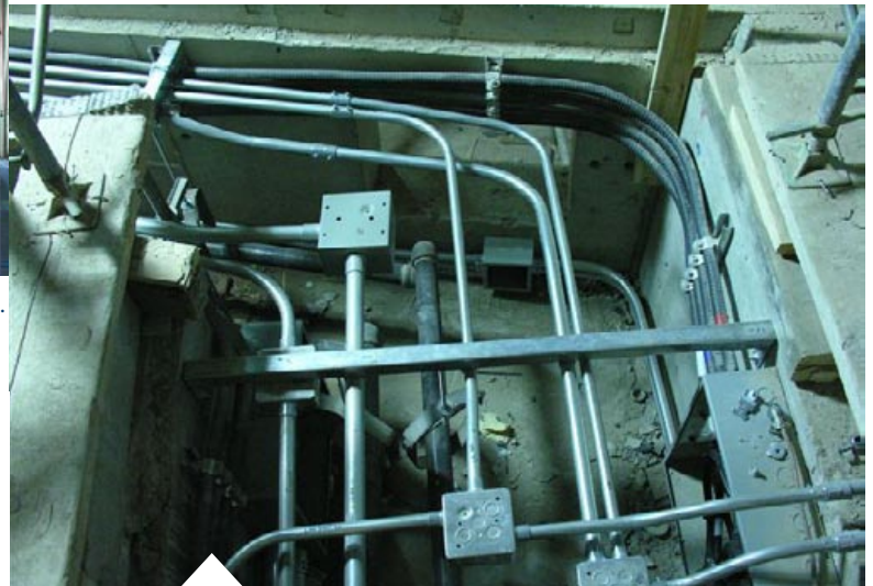
Mechanical trenches are filling up with conduit, cable, and water pipe.
