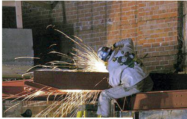
Welding steel for box seats
